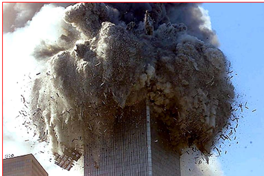
WTC Complex in New York - 11th September 2001
