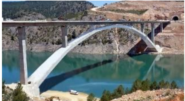
Contreras High Speed Train Viaduct. 265 main span. (Spain). Fernandez Casado SL (completed in 2009).
