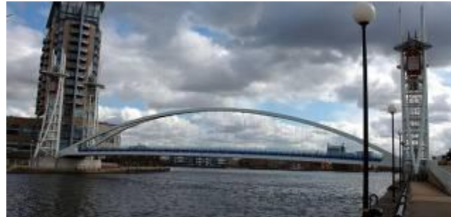
Lowry Pedestrian Lifting Bridge. 90 m main span (Manchester,UK). Fernandez Casado SL. (completed in 1999).
