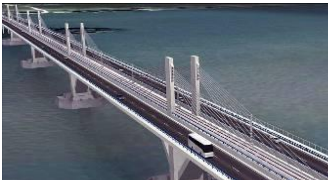
Danube Crossing. Vizny. 185m main span. (Vidin. Bulgaria) Fernandez Casado SL. (to be completed in 2011)
