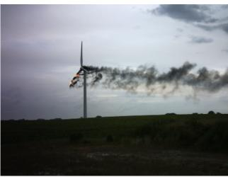
Fig. 1a+b: Fire after lightning struck a 2 MW wind turbine in 2004 (Image source: HDI/Gerling)
